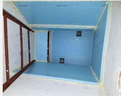
Air sealing and insulating the roof hatch
