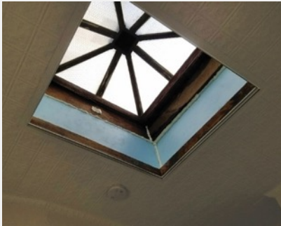
Priority tiered air sealing and weather stripping of the building
