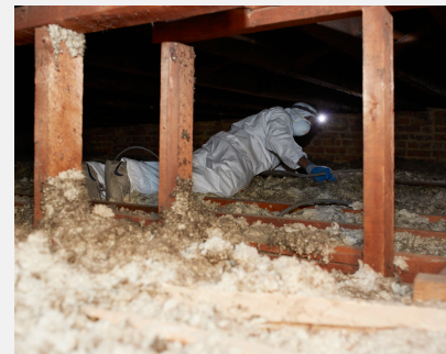
Air sealing and insulating the attic cavity
