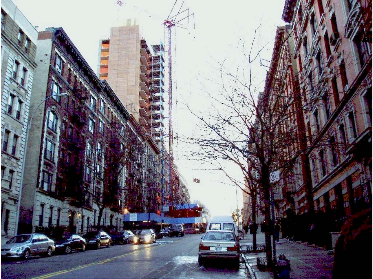
Photo B-1: “Out-of-context” building in Morningside Heights
