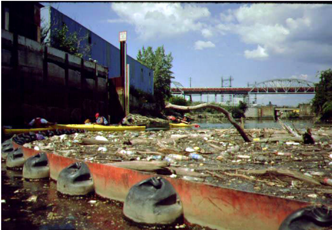
Illustration 14 – a floating boom prevents garbage from entering the Long Island Sound (and captures kayakers)
